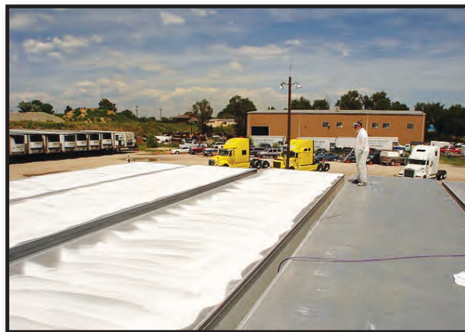
Super Therm can be sprayed over large areas or rolled onto smaller surfaces. Coating needn't be cleaned to stay effective and lasts more than 20 years.
