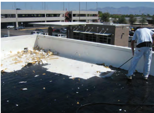
Pressure Washer Removing Elastic Coating
