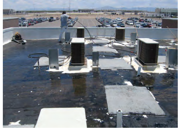
Roof During Pressure Wash
