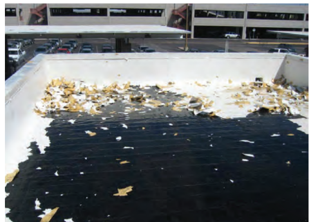
Elastic Coating removed by pressure washing
