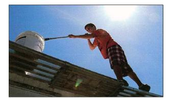
regular paint rollers, it can be applied with a paint sprayer, but *remove all filters when using a sprayer*. According to the manufacturer, the product fully "cures" in 21 days.
