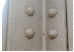
ASTM 610 Rust grade 10 M 714 Scale 10
