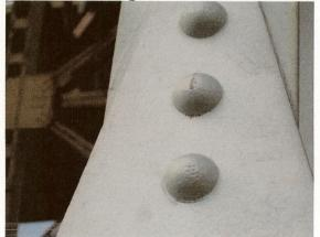
ASTM 610 Rust grade 10 M 714 Scale 10
