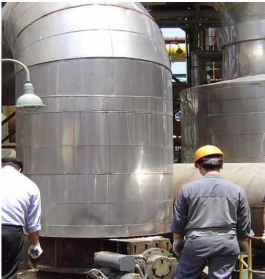
Surface temperature before HPC application: 320 C
