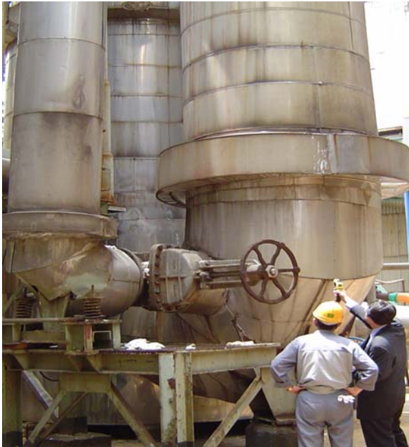
Sulfuric Acid Tank
