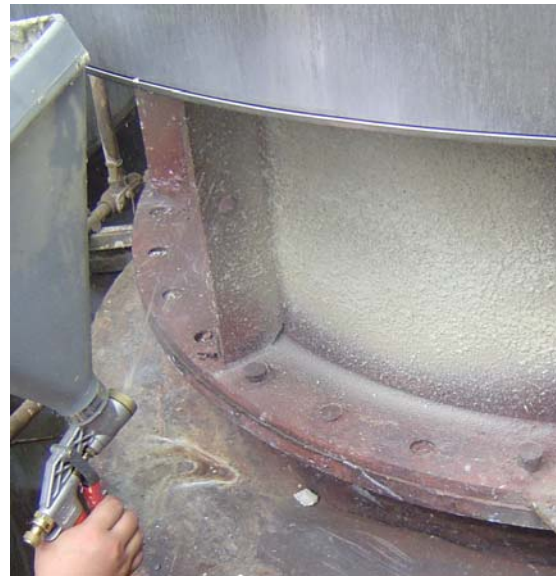
HPC application to 25 mm thickness
