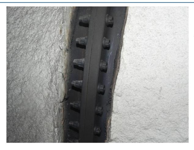
In some cases, Insulative Coatings can be applied over fiberglass or rockwool wrapped around bolts which can then be cut to expose the bolts if needed.
