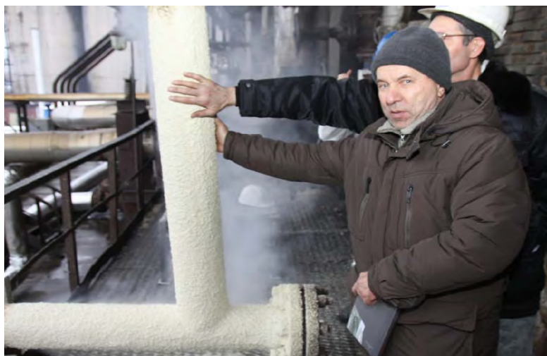
FIGURE 12: RUSSIAN ENGINEERS AT 30MM CLOSED FILM TIC WITH HANDS ON 550C PIPE DOWN TO 40C
