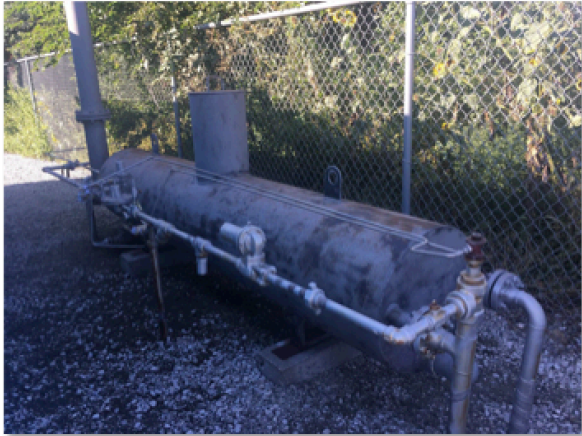
FIGURE 5: WATERBATH HEATER BEFORE AND AFTER CLOSED THICK FILM TIC
