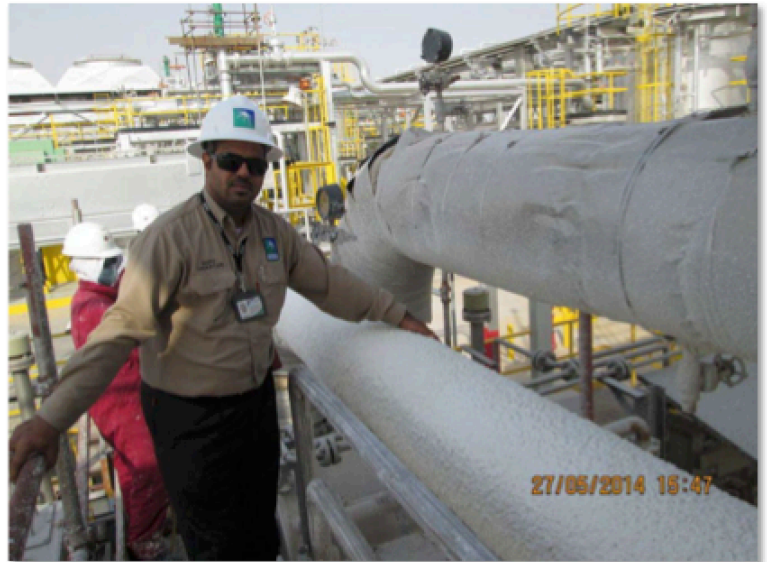
FIGURE 11: THICK CLOSED FILM TIC OFFERS PERSONNEL PROTECTION, REDUCED ENERGY LOSS AND CO2 REDUCTIONS ALL IN SITU AND WITH REAL WORLD ENVIRONMENTAL FACTORS
